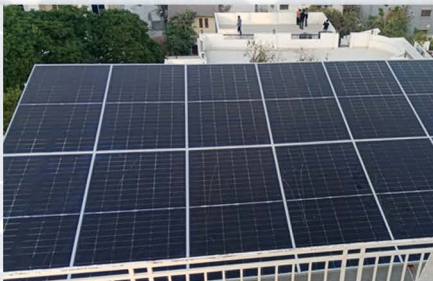
18 kw Solar Plant Installation Suncity,
