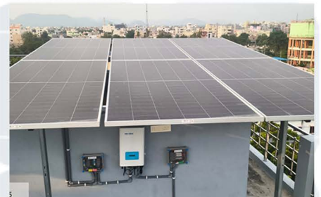
3kw Solar Plant Installation
