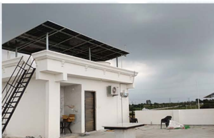
8 kw Solar Plant Installation
