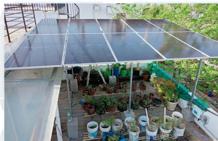
5Kw Solar Plant Installation
