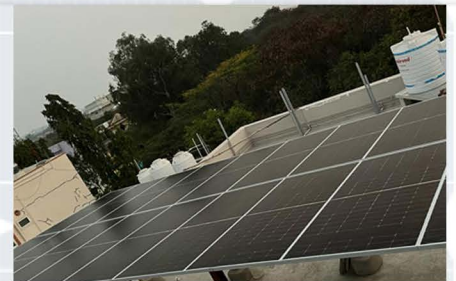
10 kw Solar Plant Installation
