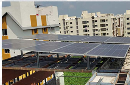
12 kw Solar Plant Installation
